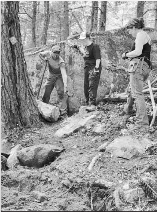
Dan, Sally, and Beth turning a steep hillside on the Lambert Trail into a trail.
