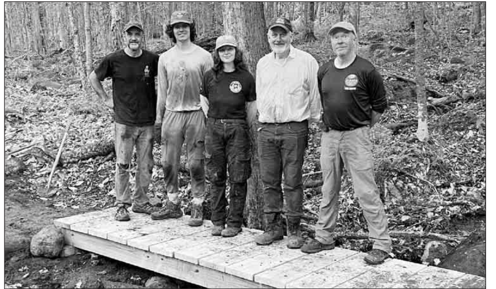
Tom Arminio, Cam Rogers, McKenna Thompson, Malcom Campbell and Scott Guay on a new bridge over an intermittent stream on the Blaisdell Trail.
